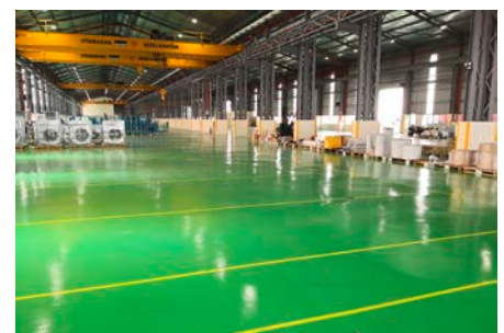
Industriehalle in Malaysia
